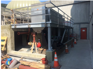
New RDT's being installed.
