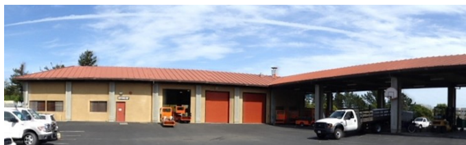
Existing maintenance building to be modified.
